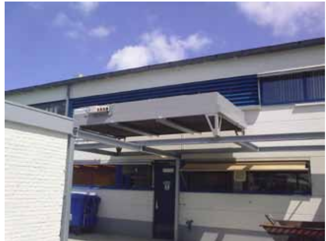
Reducing the amount of leaks in compressed air piping will result in 32 tons of CO 2 -reduction per year.
